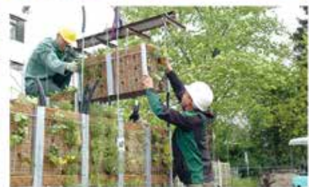
The modular principle with the pre-planted baskets quickly and easily creates green oases with function as noise barriers, privacy protection and vertical ecosystems.
